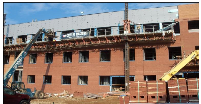
Figure 15 - View looking at east elevation. Fraco Lifts are used around the exterior to provide an efficient workflow along a large percentage of elevation at a time. Materials are lifted into place with a boom lift. Personal photograph taken by Chris Pozza.
