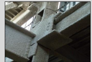
Column-to-beam moment connection.
