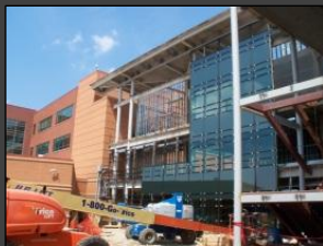
West Elevation Glass Curtain Wall.
