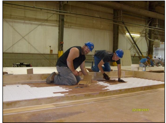
Figure 37 - Workers are able to fabricate panels comfortably in a controlled environment; increasing quality and productivity. Image taken from Gate Precast.
