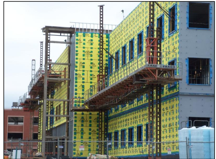
Figure 47 - View looking at the corner of the south and east façade. DensGlass can be seen in yellow, with each individual brick tie having Blueskin applied. This is a necessary step before the air and vapor barrier can be applied. Personal photograph taken by Chris Pozza.
