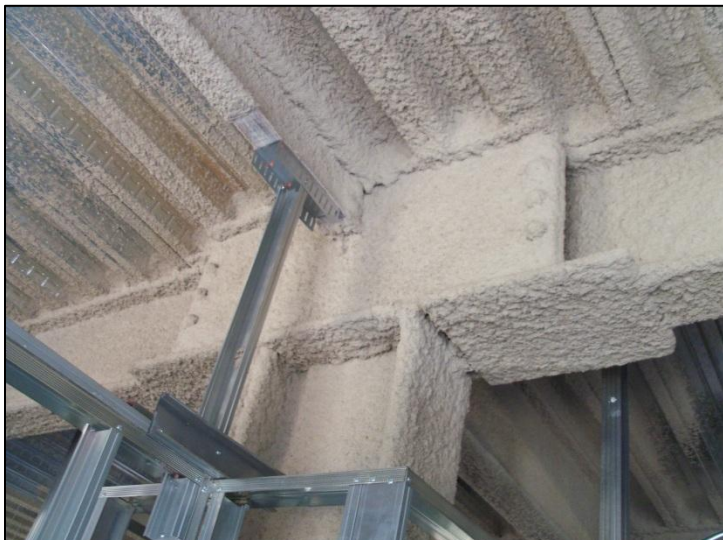
Figure 6 – Photograph of a SidePlate system which is a moment frame that connects columns to beams and girders and can be a single- or double-sided connection. Spray-on fireproofing has already been applied to the structural steel at this point of construction. Personal photograph taken by Chris Pozza.
