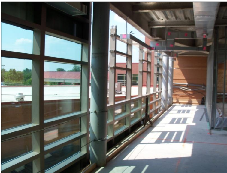
Figure 17, left – Interior view of west elevation curtain wall system under construction. Personal photograph taken by Chris Pozza.
