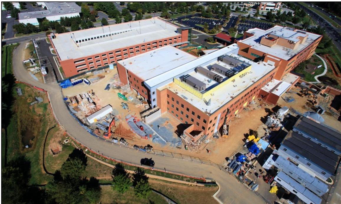
Figure 1 - Progress photo of the addition taken in September 2012. Image courtesy of DPR.
