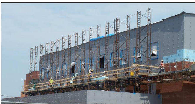
Figure 14 - View looking at southwest elevation. A MasonKing lift is required in areas where work is done above rooftops. These lifts have to be simultaneously cranked by hand on each side to be lowered or raised. Personal photograph taken by Chris Pozza.
