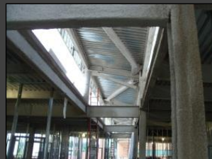
Clerestory spanning 3 rd floor addition.
